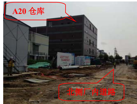
拟建变电站北侧
